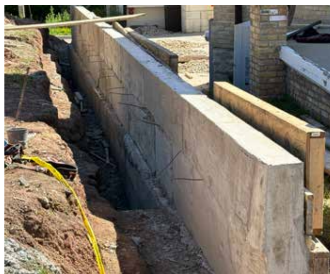
New Retaining Wall
