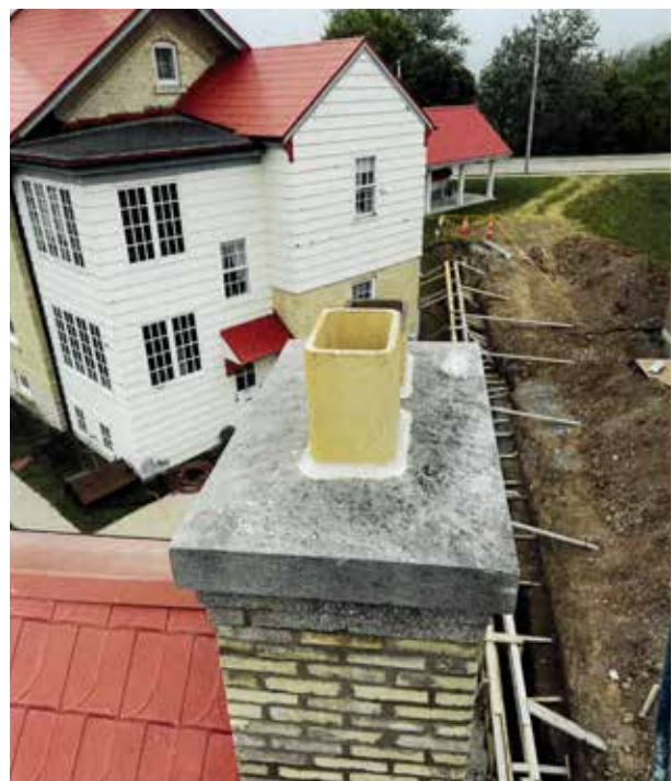
2026 Capital Improvements - Chimney Rebuild and New Concrete Wall
