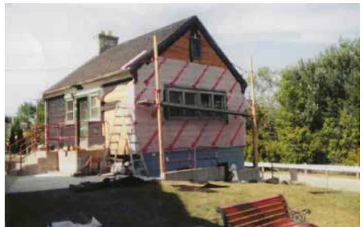
2002 Renovation of Generator Building
